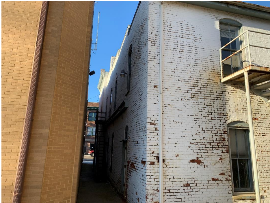
View of D side of structure
