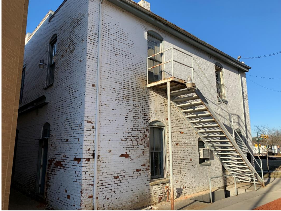
View of C side of structure
