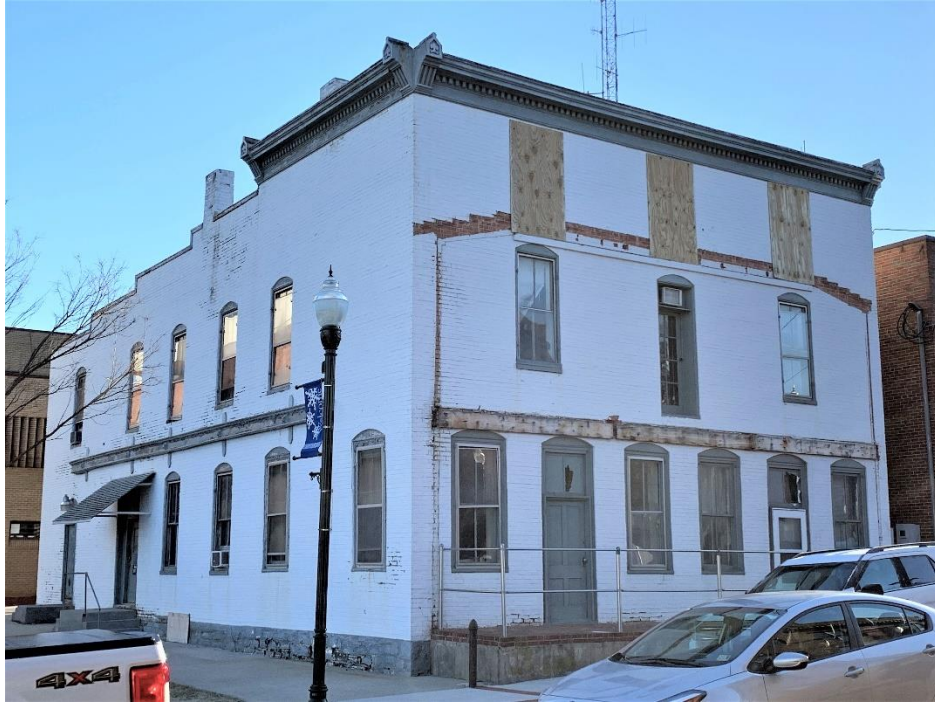
View of A side of structure
